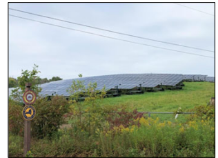
2.7 MW Community solar array on Town of Elbridge landfill
