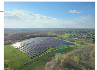
5.7 MW Community solar array on Town of Manlius landfill
